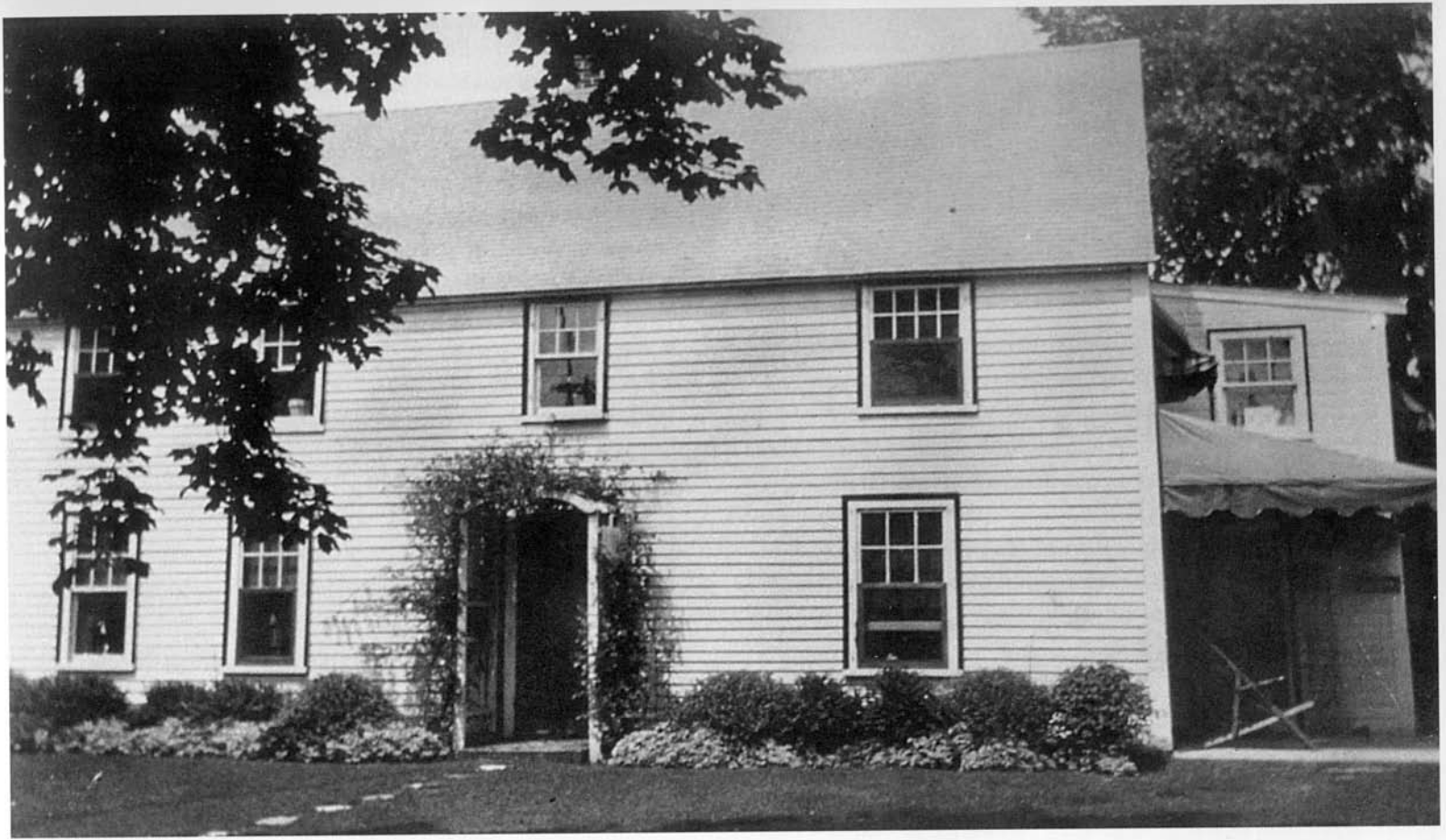
The Whittemore house, at one time the home of Fitz H. Lane, was built circa 1700 of plank frame construction. Courtesy of Sharon Howard.
